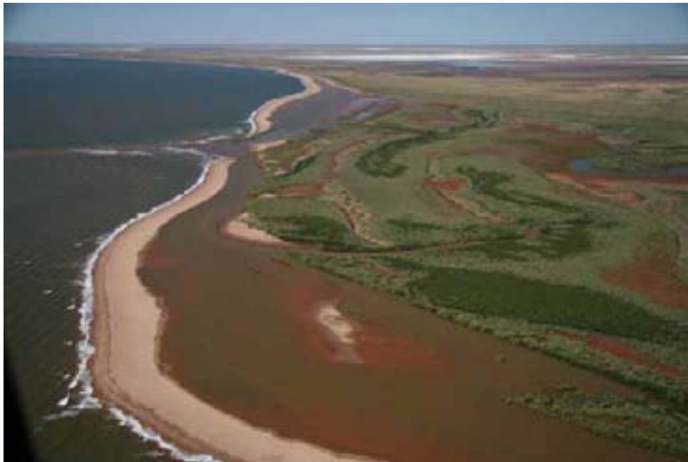
Plate 5-1 Aerial view of the north-eastern lagoon of the Ashburton Delta facing east. The proposed pipeline route is in the upper lagoon in the photo.
