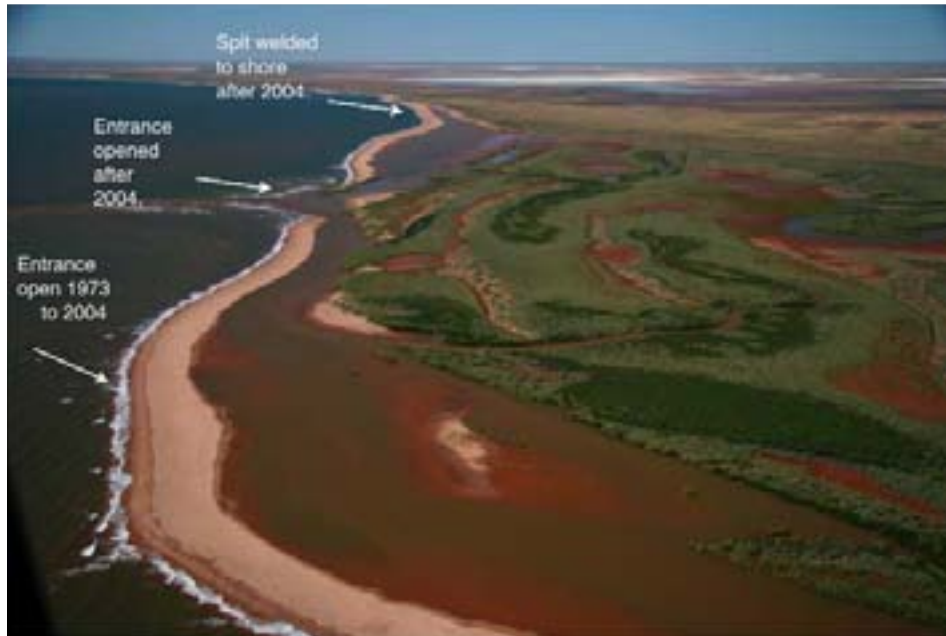
Plate 4-2 Entrance Point looking east
