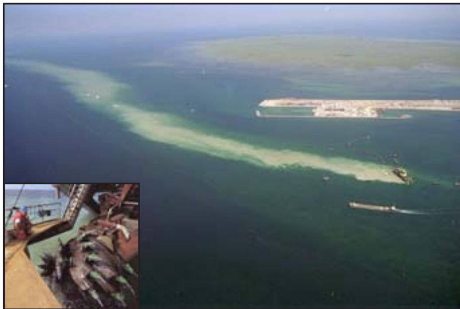
Photo B.1 Large sediment plume from cutter suction dredger Castor, 7 August 1997. Inset shows cutter head
