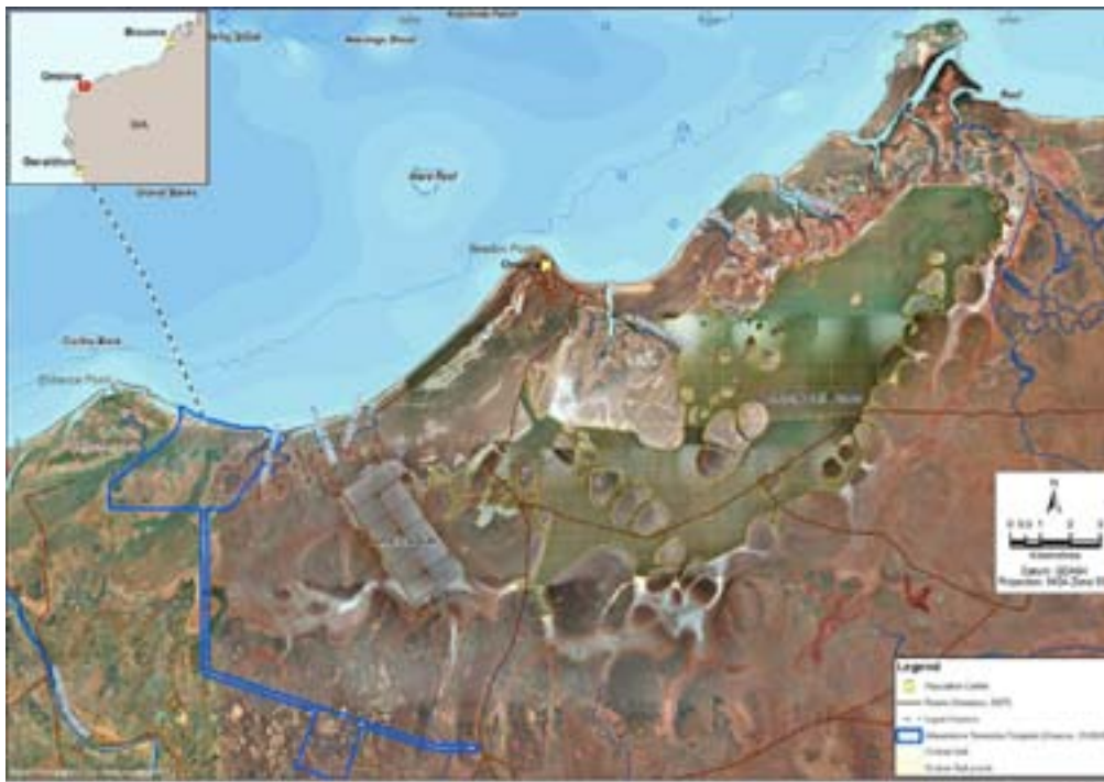
Figure 3-2 Onslow salt ponds and onshore Project area
